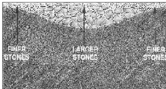
*Slurry surfacing shape correction work (photo courtesy Pioneer Road Surfaces)*
