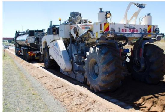
**Fig 2** Foamed bitumen stabilisation process
