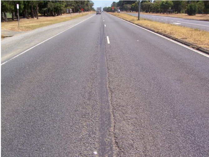
Figure 3. Stripping of seal from overlapped fabric placed without additional binder allowance
