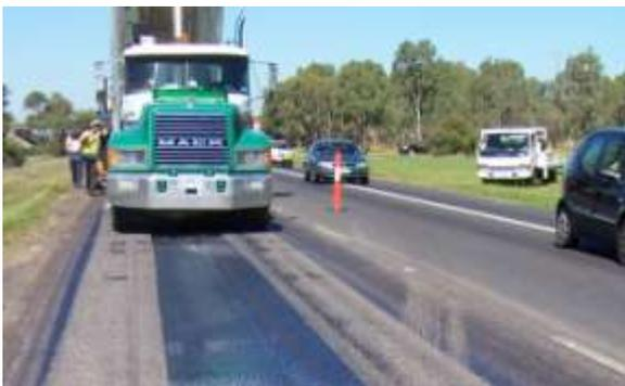
Figure 2 Pick-up of tack coat on dusty milled surface
