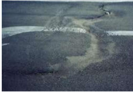
Figure 3 Asphalt slippage failure on concrete pavement
