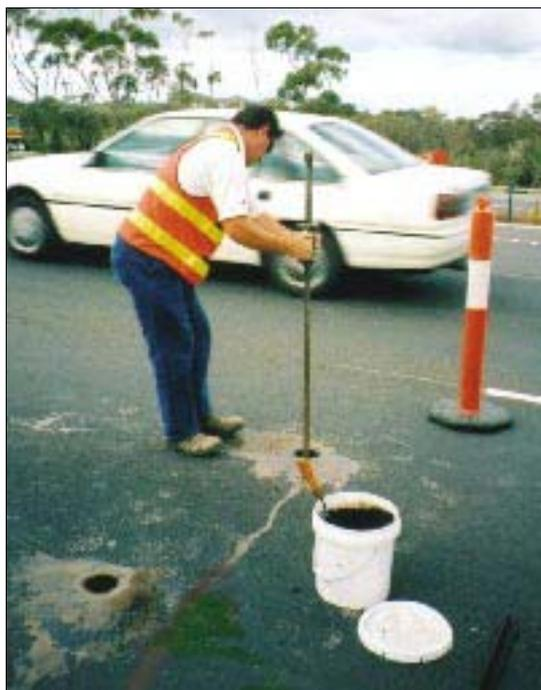
Figure 3: Reinstating core hole slide hammer
