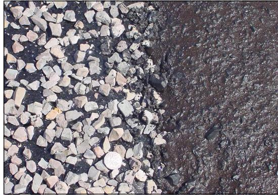
Figure 4. Sprayed seal (left) and finished slurry surface (right)
