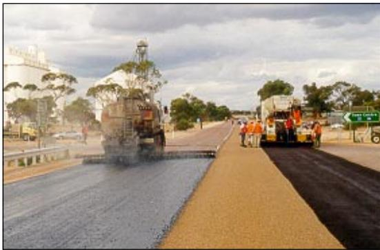
Figure 3. Work in progress showing sequence of binder aggregate and slurry
